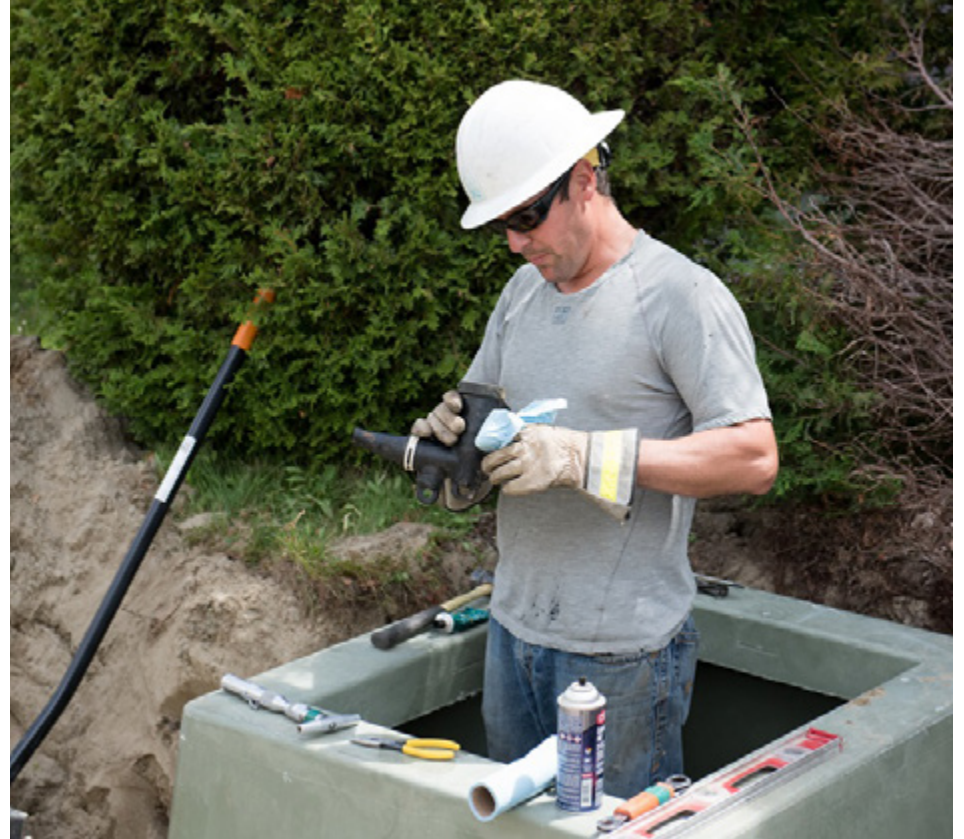
If you think you might need new or upgraded electricity service, even months from now, please contact VEC as soon as possible so we can be sure your service is available when you need it. Above, VEC Lineworker First Class Alan Esposito works on a job site this summer. Photo VEC/Kevin Goddard.
